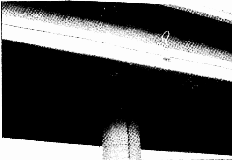
b. View of the Underside Showing Complete Absence of Damage and One of the 26 Accelerometers Installed at the Site. The Peak Horizontal Ground Motion Component Recorded at the Free-Field Site Adjacent to the Bridge Was 0.33 g.
