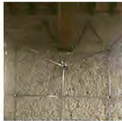
Detail of the link to the R/C kerb around a wooden truss.
