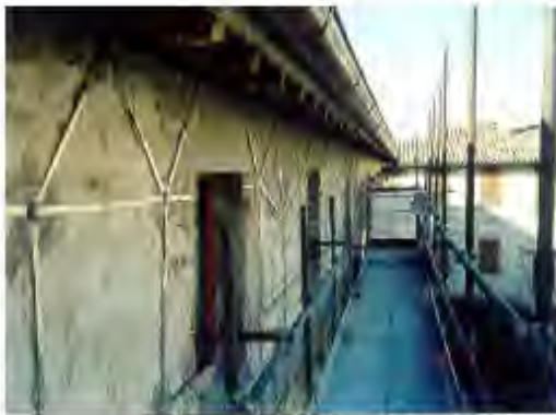
Application of the CAM method to the seismic improvement of a masonry apartment building at Sigillo (Perugia) (filmed during works in December 2000).
