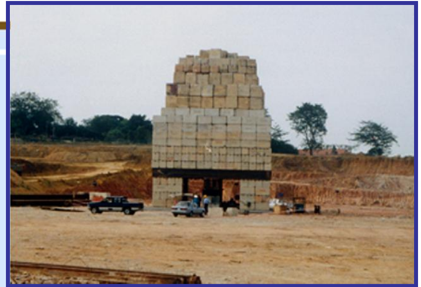
300 ton Surcharge System
