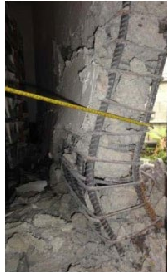
Wall lateral buckling (Source: "Seismic Design of Reinforced Concrete Buildings" by Jack Moehle)
