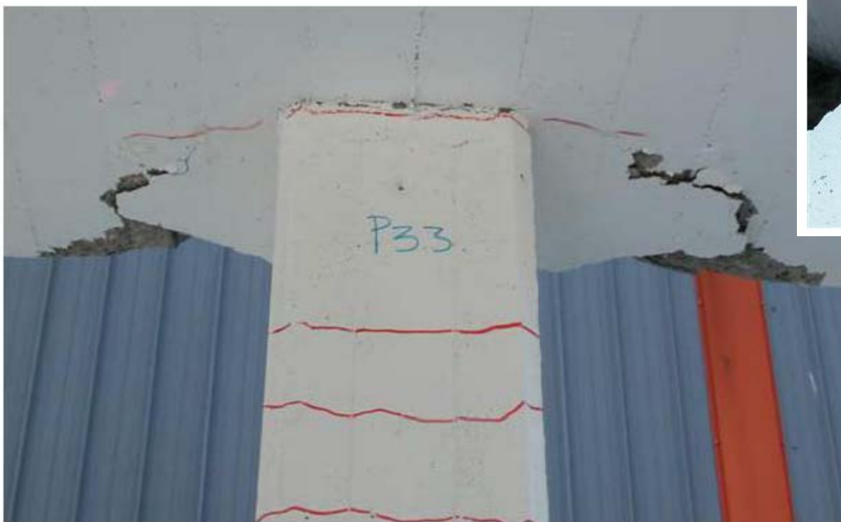
2. Floor 3 (below): detachment of the slab above column P
