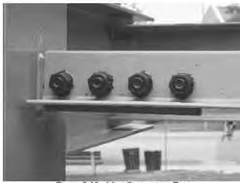
Figure 7-18. Misc. Connection: Truss Column C2 / Truss B7
