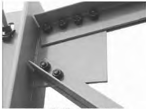
Figure 7-17. Misc. Connection: Truss Column C2 / Truss B7
